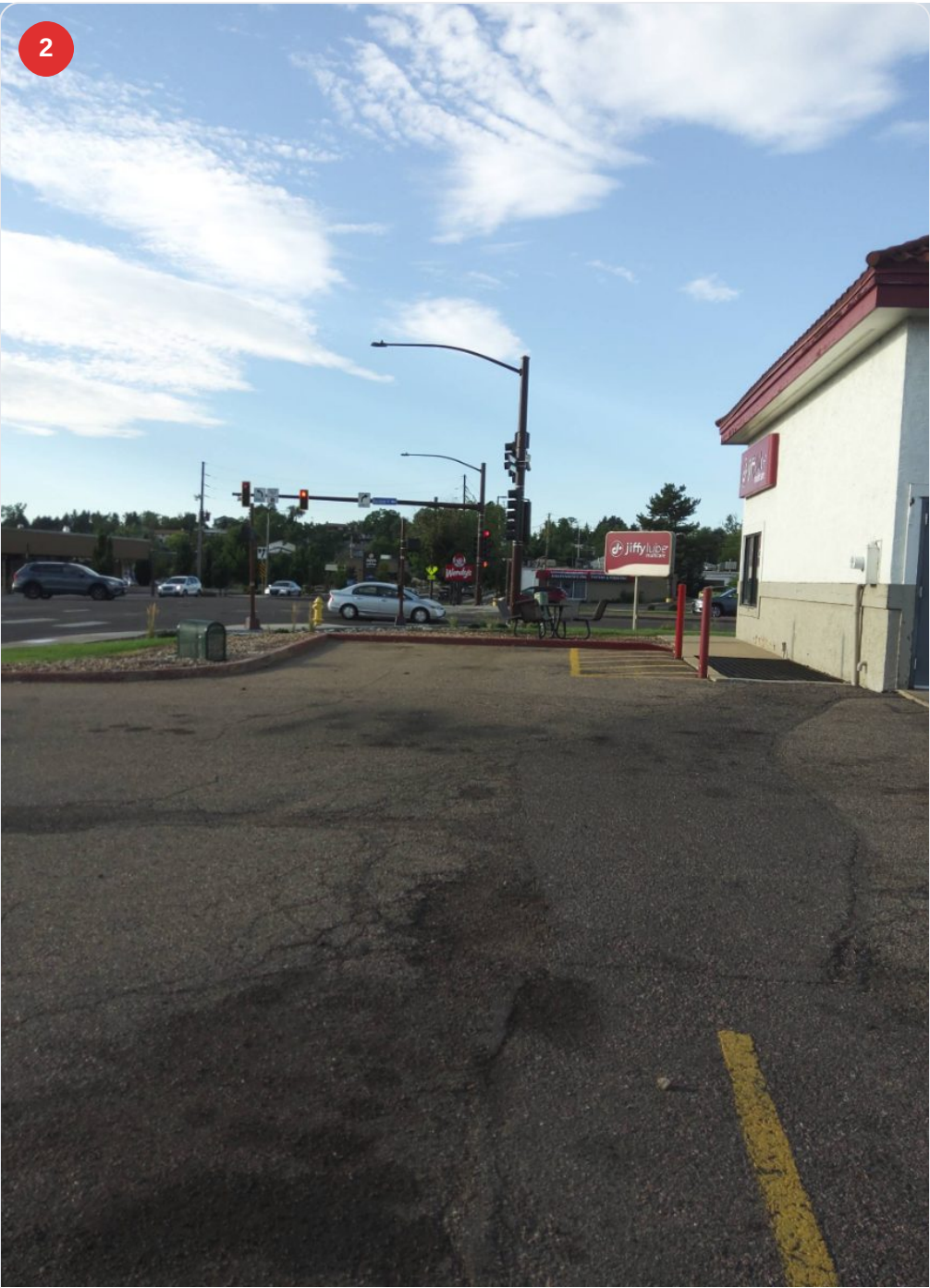
📍 Unit 5805 Independence St 81 Curb Striping 5 Parking Stall 3 Arrow 11 Bollard Curb Striping — 81 LF · red · Parking Stall — 5 · Arrow — 3 · Bollard — 11 Aug 24, 2026, 7:56 AM
